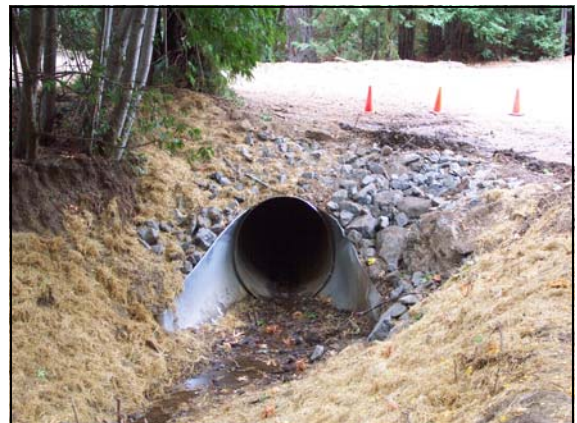
Undersized culvert was removed. The proper culvert was then installed and set at grade. The flared outlets will prevent the culvert from plugging.
